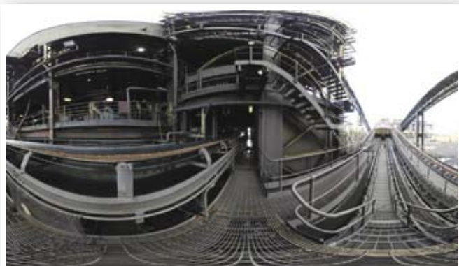
Unwrapped spherical of the manganese plant showing conveyors transferring material
