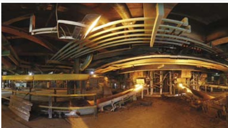
Unwrapped SiteSee of the dangerous slag tapping area (see www.aamgroup.com/siteseesafety.cfm for an interactive version of this example)
