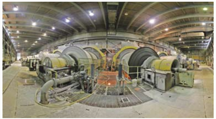
Unwrapped SiteSee of the mill building
