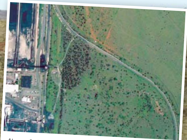
Above: Ortho image of the rail expansion project
